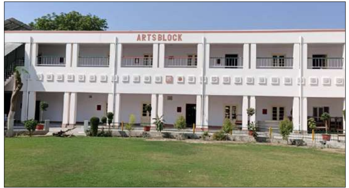
Block in-front of Principal Office
